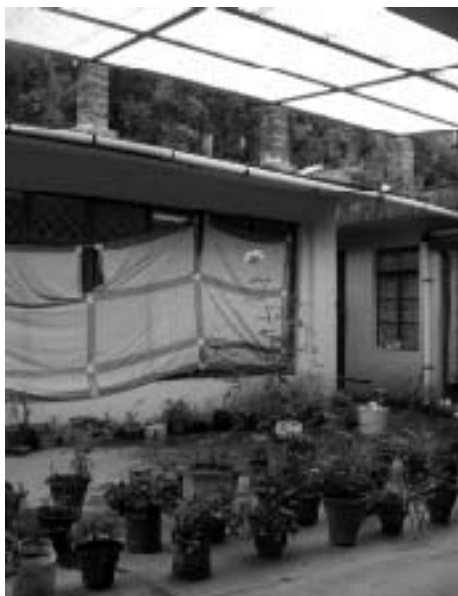
The newly covered rooftop area
