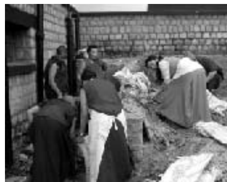
Nuns and lay students help with construction during regular work periods
