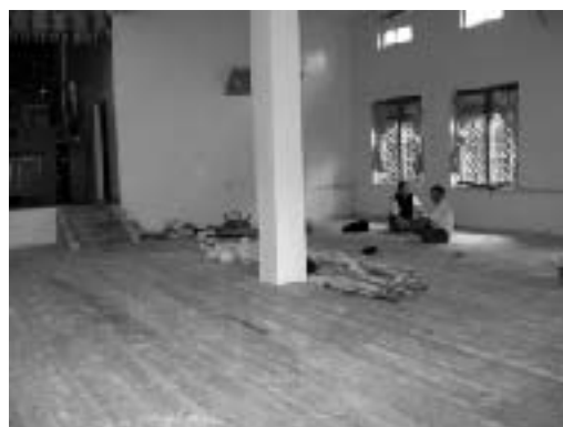
The new wooden floor nearly complete
