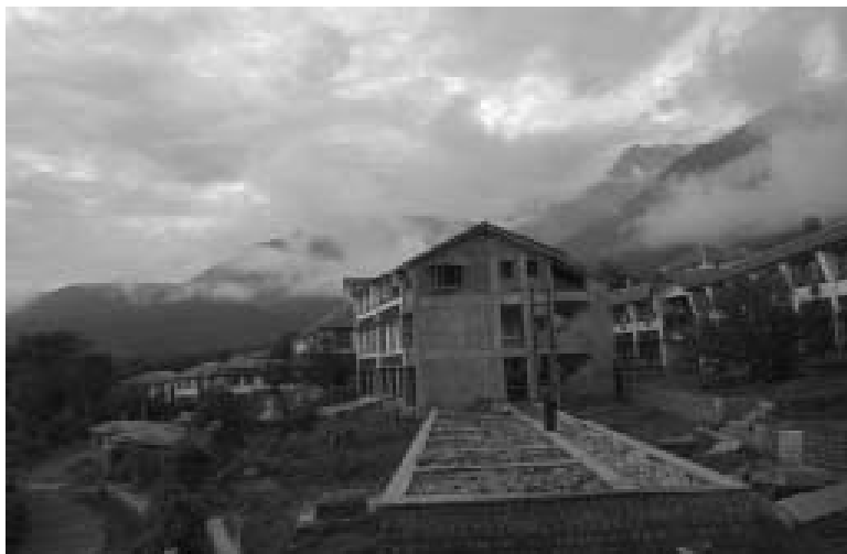
Completed classrooms of the
