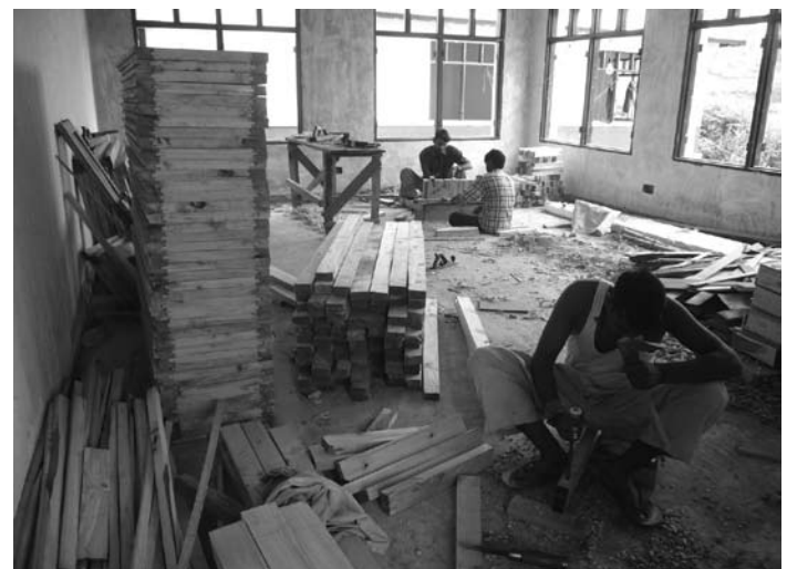
Carpenters making window shutters
