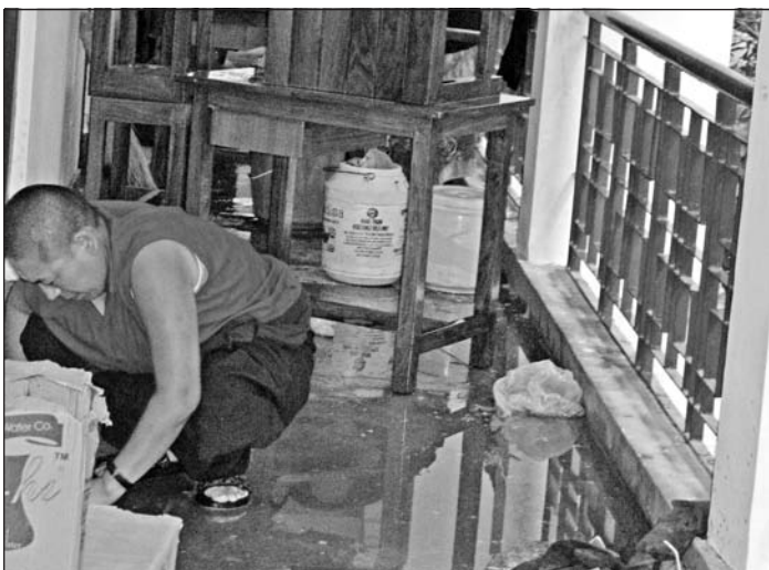
Cleaning a room before moving in
