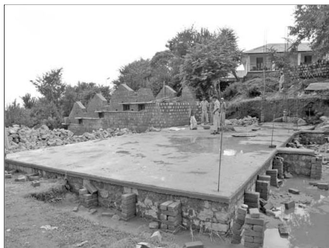
Solar bath house
