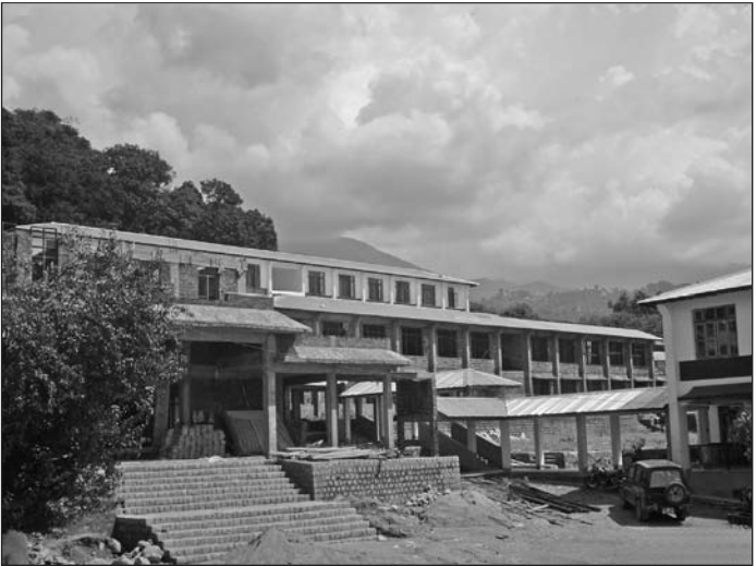
View of the first and second housing wings and roofed pathways
