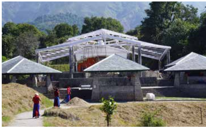
Roofing for the debating courtyard
